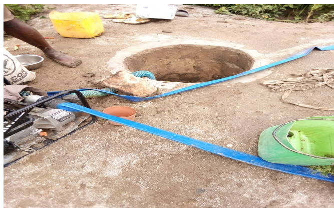
Figure 4. Constructed shallow well for motorized pump irrigation
