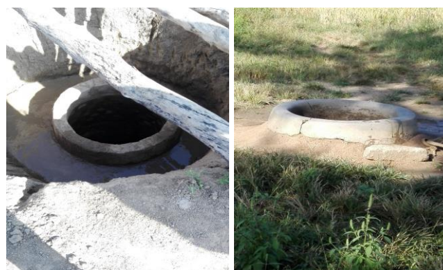
Figure 5: A Well Under Construction and a Completely Developed Well
