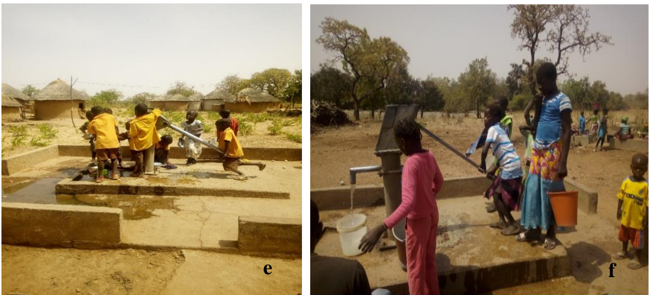
Plate 3. Children Playing with the Handles of Boreholes; Causing Breakdowns at Gurugu (e) and Aseyili (f) communities
